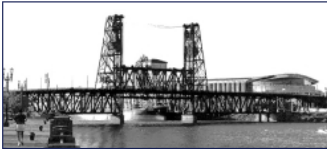
Portland's Steel Bridge
